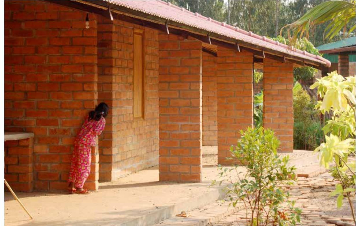
1. Community Centre in Oudong (Cambodia) for habitat for Humanity. The building was designed placing particular attention to the way it relates with the surrounding.
