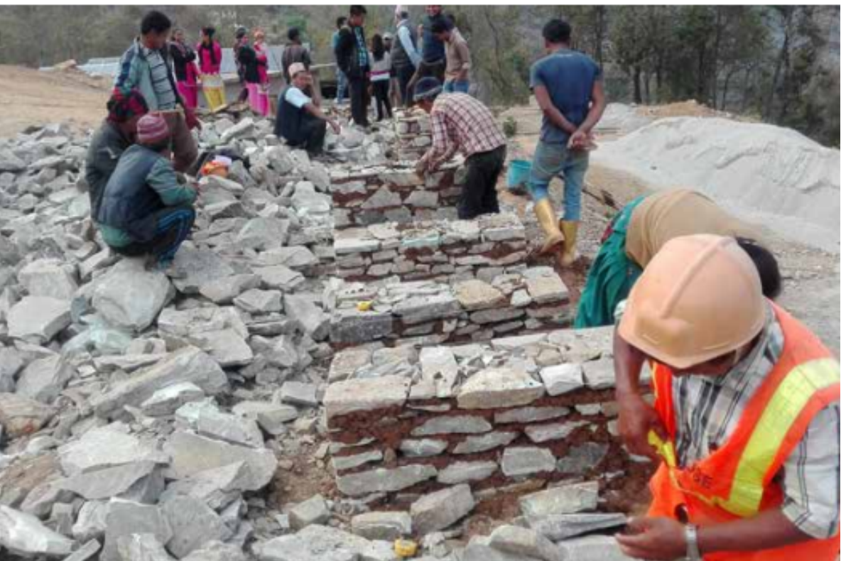
Builder's training for earthquake prone construction, Nepal 2016
